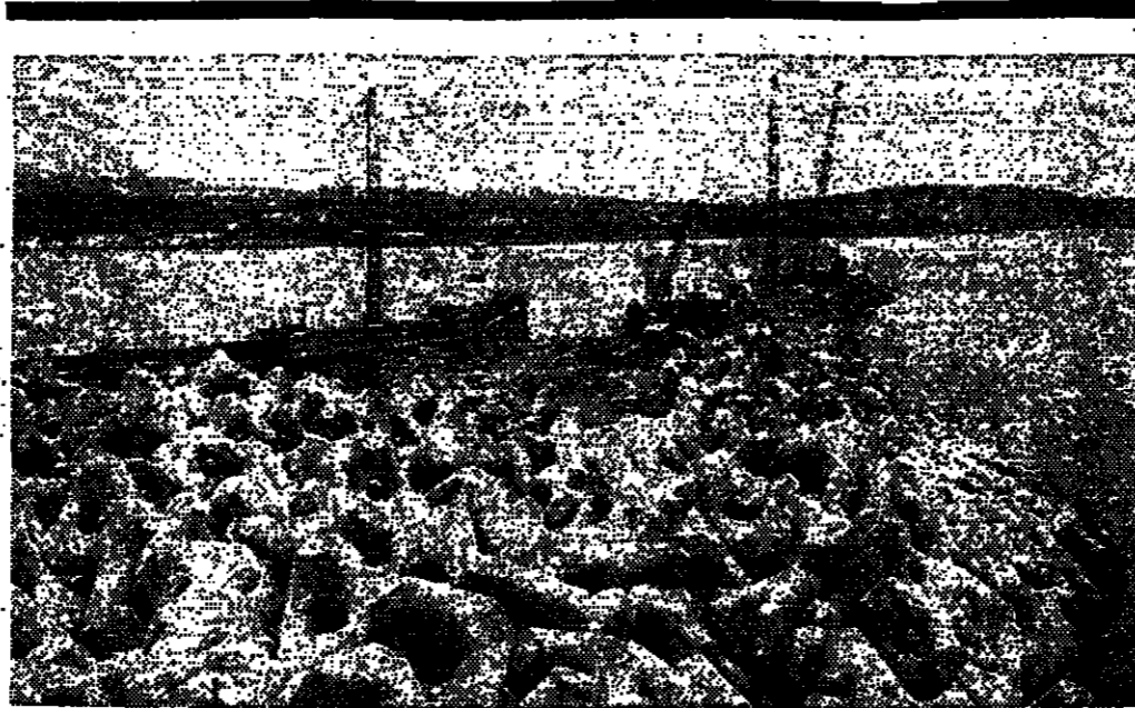
One of the island's major capital works projects is the extension of the Battery Pier Breakwater at the harbour of Douglas. Contractors French Kier Construction are looking for completion by next December. Picture shows the concrete stabilisation units ready for positioning on the rubble base
